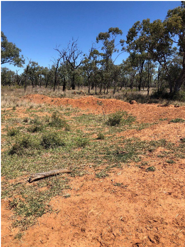
Left. Woa boy diverts water flow off roadways and distributes across the landscape. Right. Area of previously bare land has recovered after two wet seasons.
