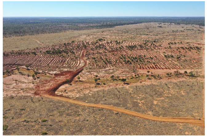
The completed project showing earth dam, spreader channels and ripped bare areas.
